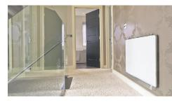
The heating technology used by Logicor in its systems is based on far infrared energy, which uses pulsed and phased electricity controlled by algorithms to make it extremely energy efficient. It doesn't heat the air but gives off infrared energy that heats the structure, furnishings and people within
